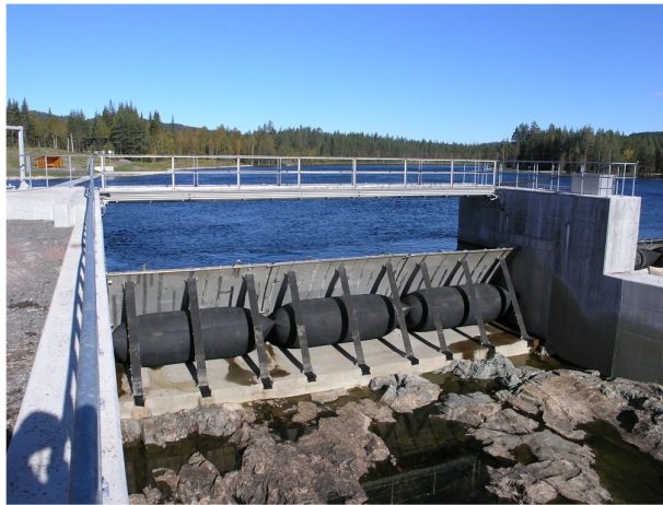
Figure 3. Flap gate with air bags (Obermeyer)
