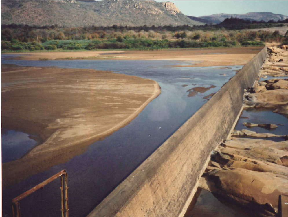
Figure 1. Typical river weir which is totally silted up.
