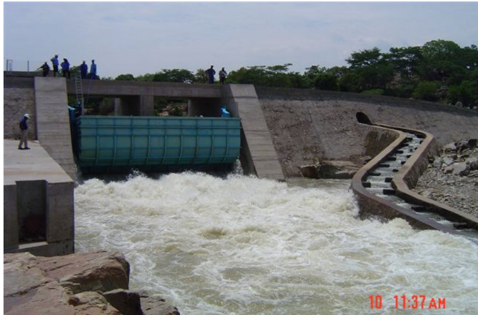
Photograph 5 TOPS Scour Gates on the Runde River, Zimbabwe
