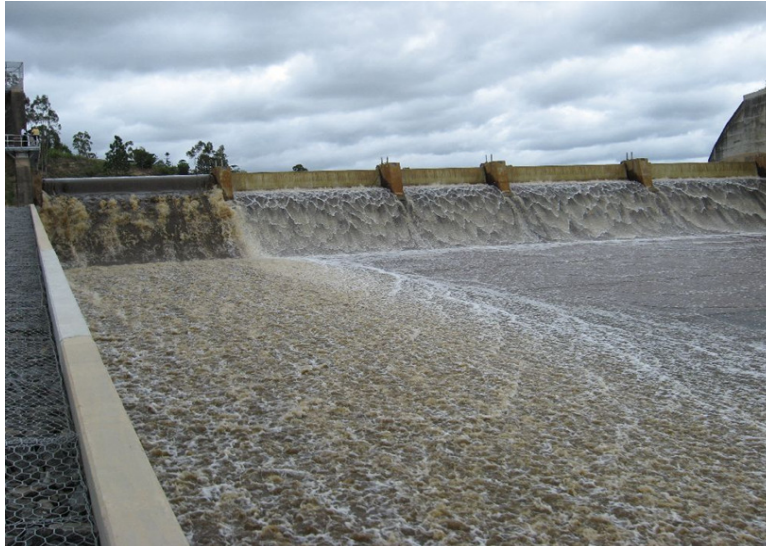
Photograph 2 2m high Crest Gates, Australia
