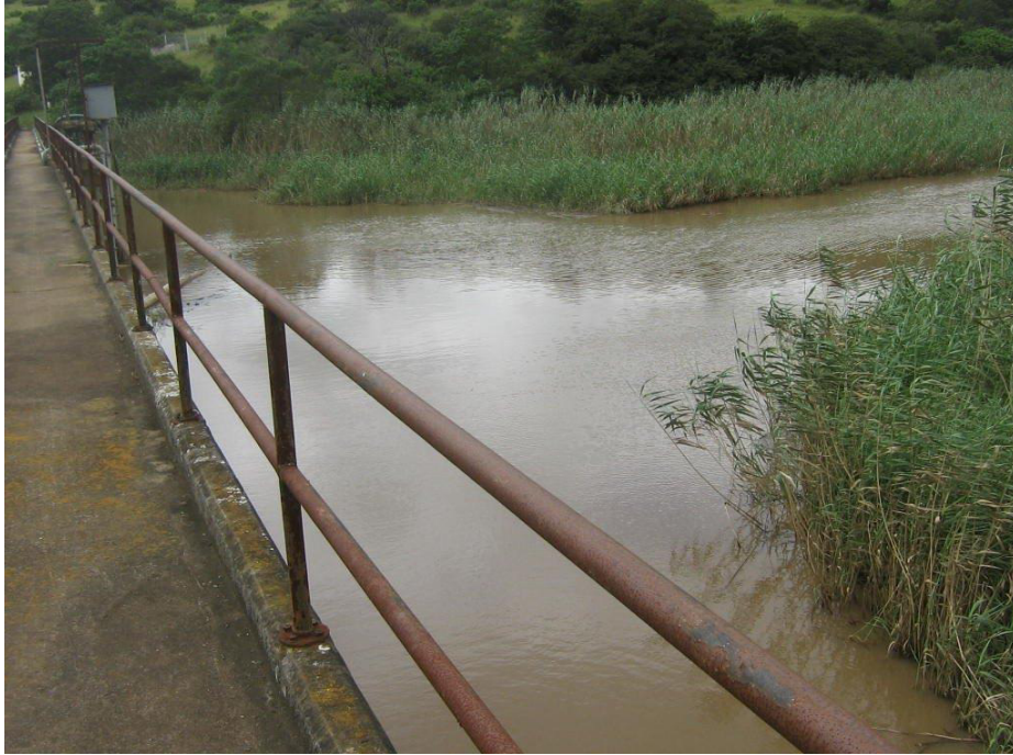
Photograph 7 30 m high Dam in KwaZulu Natal totally silted up!
