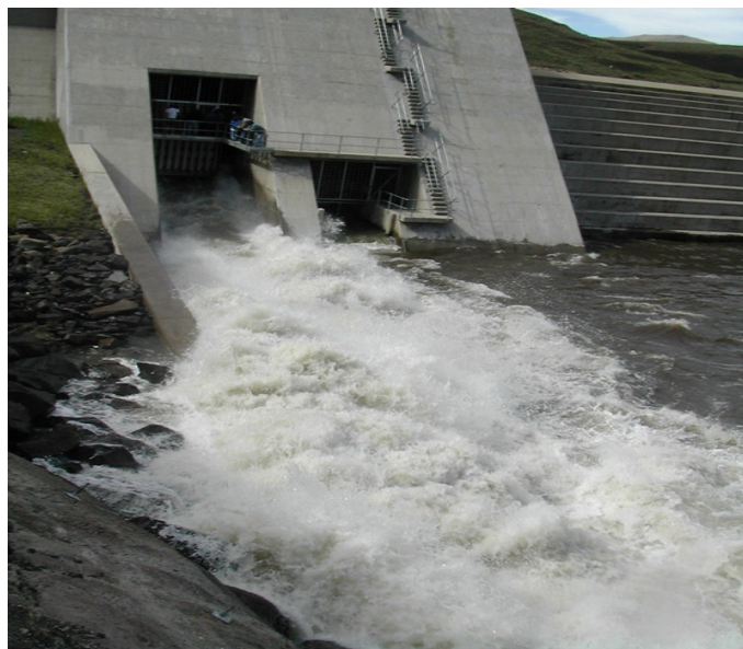
Photograph 3 Large Scour Gate under 10m head at Matsoku weir, Lesotho highlands Water Scheme
