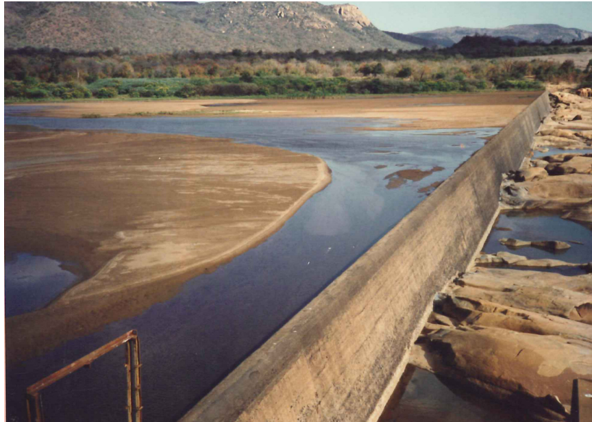
Photograph 4 Typical river weir which is totally silted up. Note the degradation of sediment on the downstream side, which is also an ecological concern.
