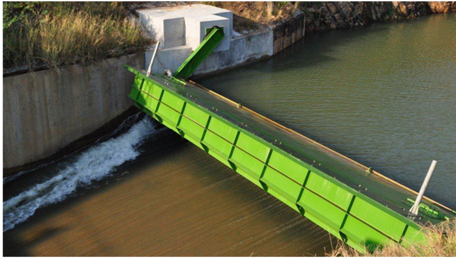
Figure 5. TOPS gate open to pass flood water on Mnjoli dam, Swaziland
