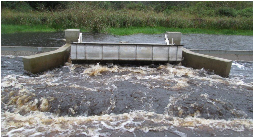
Figure 8. TOPS estuarine gate on the Karatara river at Sedgefield, South Africa
