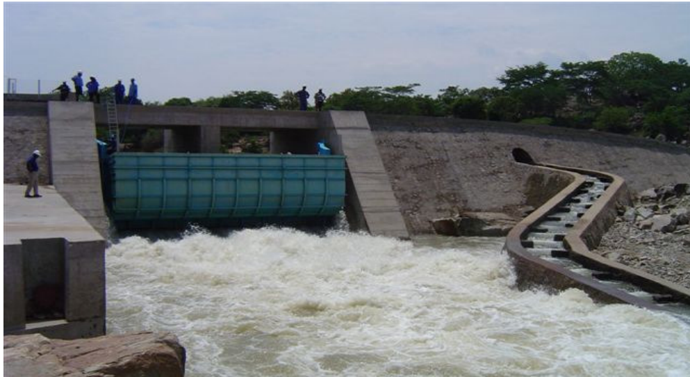
Figure 7. 4m high TOPS gate, an effective scour gate on the Rundu river weir, Zimbabwe
