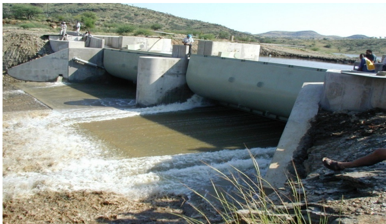
Figure 6. Avis Dam Namibia: 3m high TOPS gates on a side channel spillway
