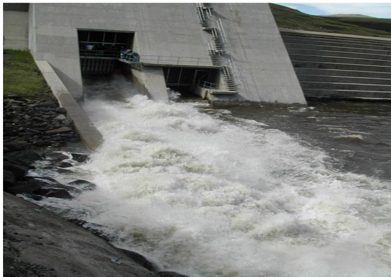
Figure 11. Large Scour Gate at Matsoku River weir, Lesotho highland Water Scheme
