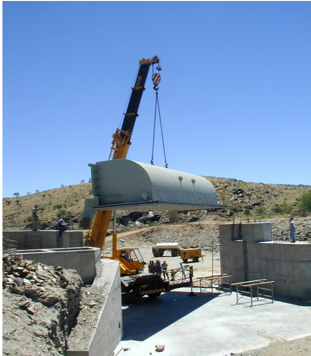
Gate lifted complete into position
