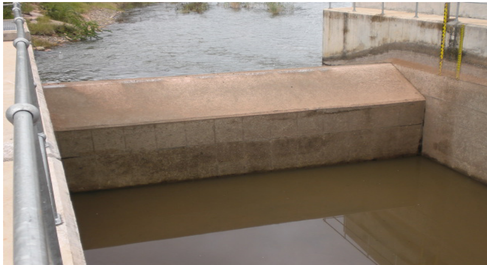
Photograph 3 Crump weir for flows up to 12,5m 3 /sec
