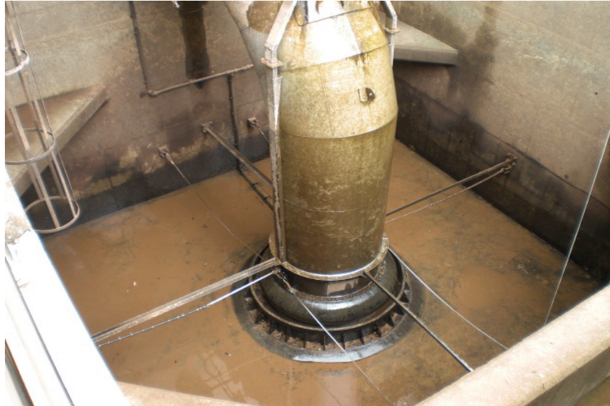
Photograph 2 1600NB Diaphragm Valve
