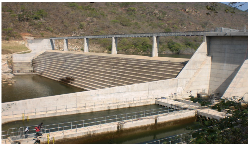
Photograph 1 Regulating weir with DV chamber and discharge channels in foreground
