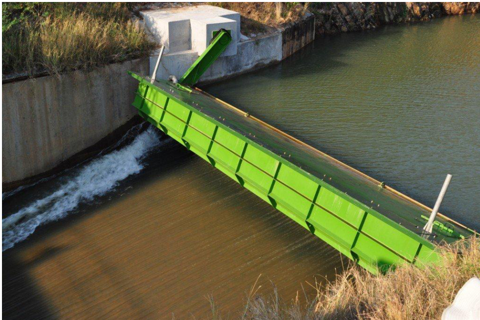
Photograph 2: Mnjoli dam service spillway TOPS gate open to pass flood
