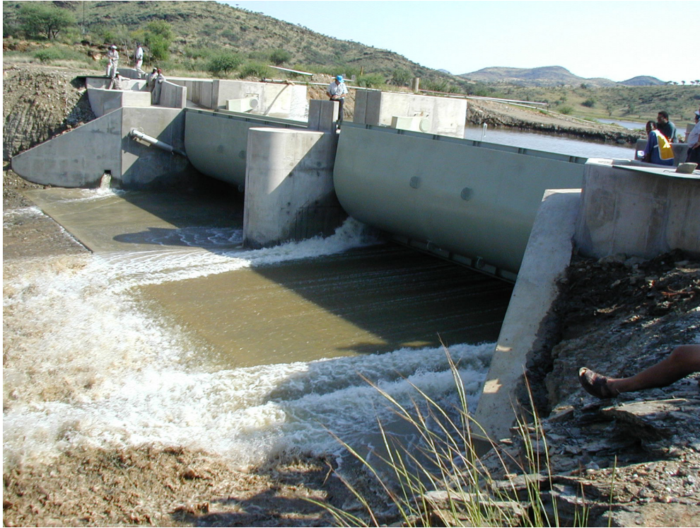
Photograph 1: AVIS dam, Namibia: Two TOPS gates used to retain FSL in side channel auxiliary spillway.
