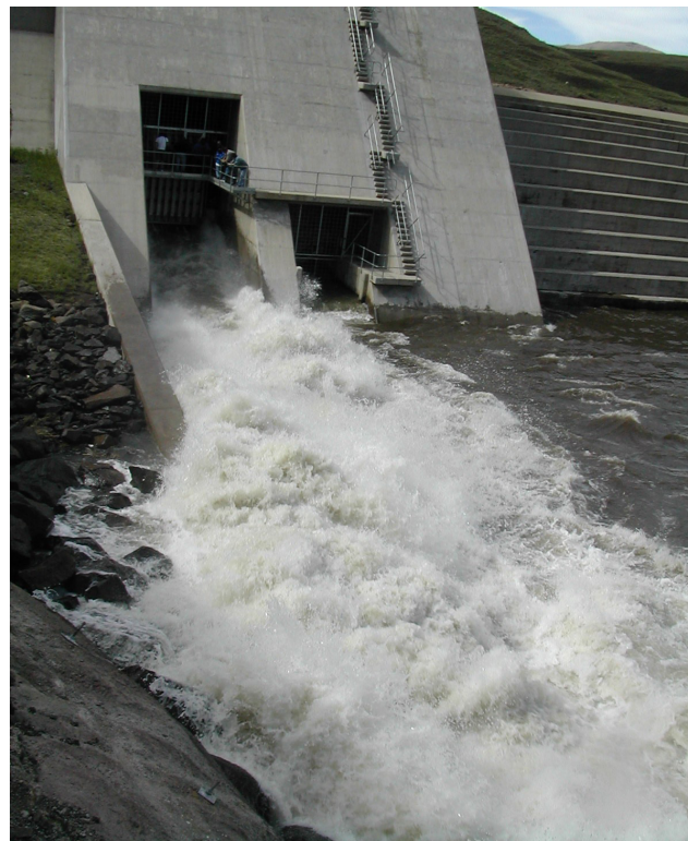
Photograph 3: 60m 3 /sec discharge from a 3m wide x 2m high scour gate: Matsoku weir, Lesotho
