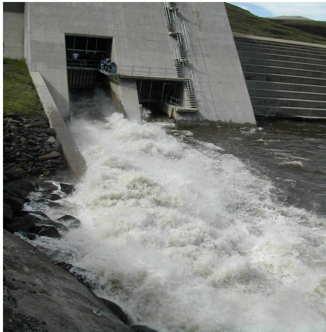
Matsoku Weir scour gate. This large scour gate keeps the forebay to the tunnel to Katse Dam relatively free of sediment. This opens frequently.
