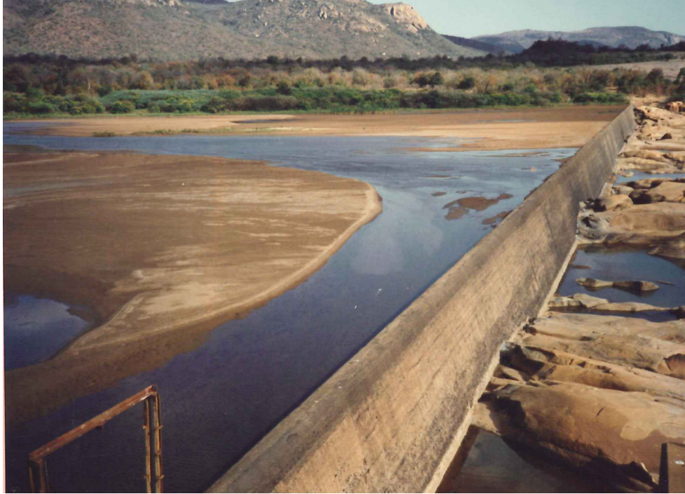
Photograph 1 Typical river weir which is totally silted up. Note the degradation of sediment on the downstream side.
