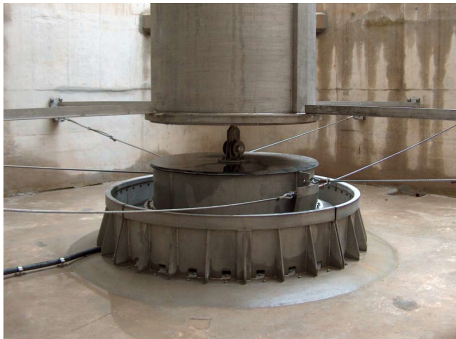
Photograph 1: Diaphragm Valve
