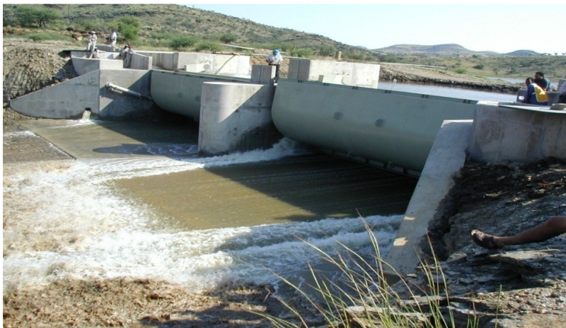
Figure 7. Avis Dam Namibia: 3m high TOPS gates on a side channel spillway
