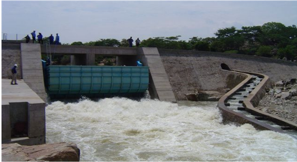
Figure 8. 4m high TOPS gate, an effective scour gate on the Rundu river weir, Zimbabwe
