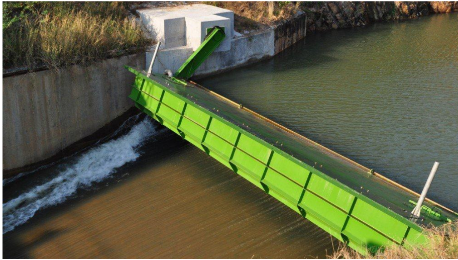
Figure 6. TOPS gate open to pass flood water on Mnjoli dam, Swaziland
