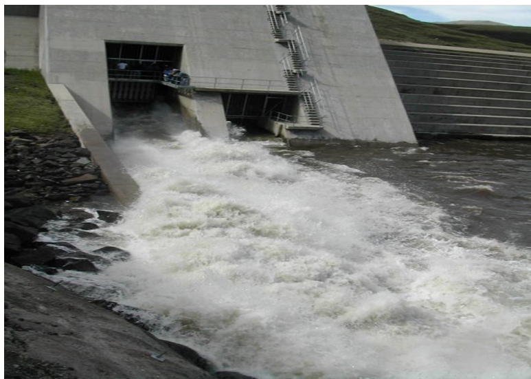
Figure 12. Large Scour Gate at Matsoku River weir, Lesotho highland Water Scheme
