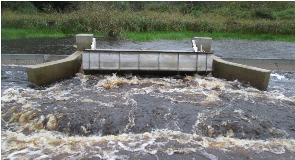
Figure 9. TOPS estuarine gate on the Karatara river at Sedgefield, South Africa
