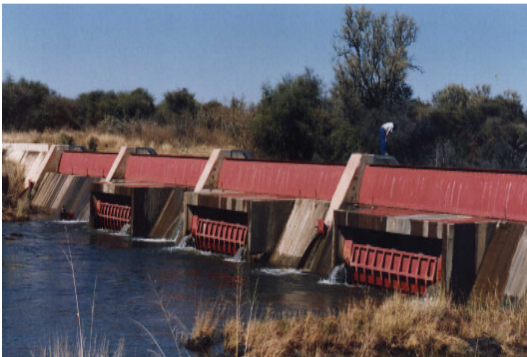
Figure 4. Scour gate operation
