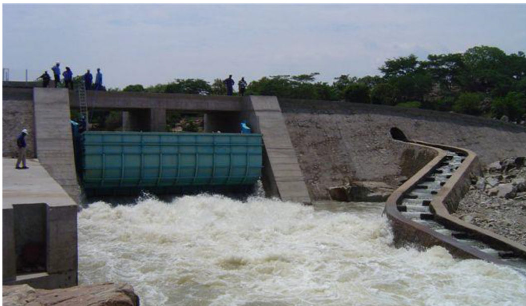
Figure 3. Runde Weir TOPS gate as an effective barrage gate to remove sediment
