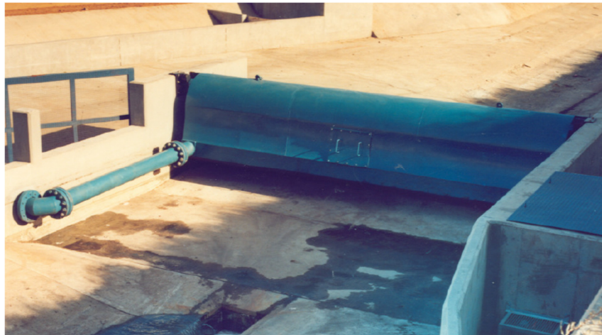
Figure 7. Robinson canal regulating gate
